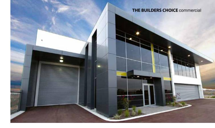
The dramatic and modern street façade is complemented by curtain wall glazing, sun shading, louvres and composite aluminium cladding systems.
